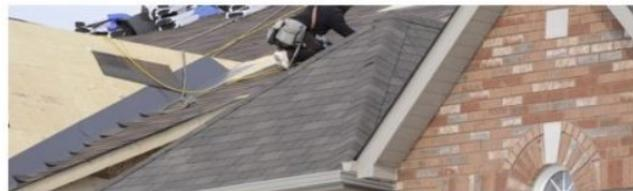
Building a roof has two phases. The first, roof construction, deals with the structure of the roof. Building the rafters, installing the fascia and more are all considered roof construction. The second, roof installation, deals with the "exterior" of the roof. Things like laying felt and shingles or rolling TPO sheets are considered roof installation. Lucky for you, Overhead Solutions employs experts in roof installation and construction.
